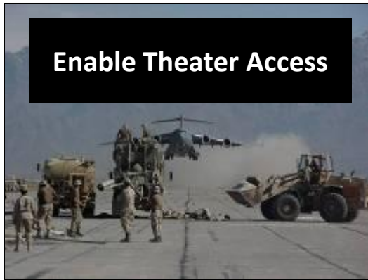
Rapid Airfield Construction
